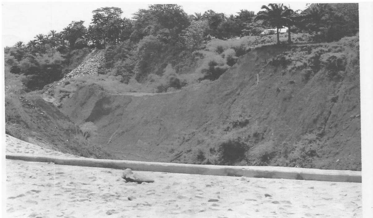
Plate 2: An Erosion Site Undergoing Control with Revetment Construction in Awka-Etiti (In the Nnewi Drainage Area). Source: The Researcher, February, 2018.
