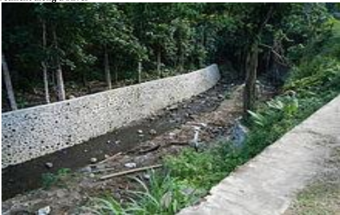
Fig. 4. Revetment along a River
